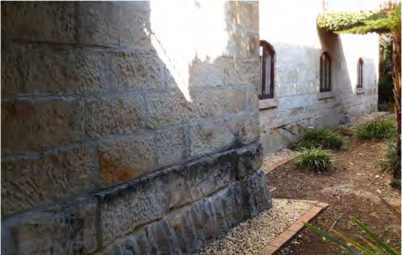
Image 2.9. Lower north façade, showing the lowest course of sandstone “bricks” as actually bedrock. It appears that the bedrock, sandstone, ground floor of the building was excavated c.2003 to expand the interior volume of the building to allow for five floors of living areas. (Source: BHHH, 2018)
