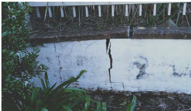
Image 6.3. Cracks sighted in 2020 in the rendered brick plinth section of the northern boundary retaining wall between the carpark and the railway reserve. (Source: BHHH, 2020)
