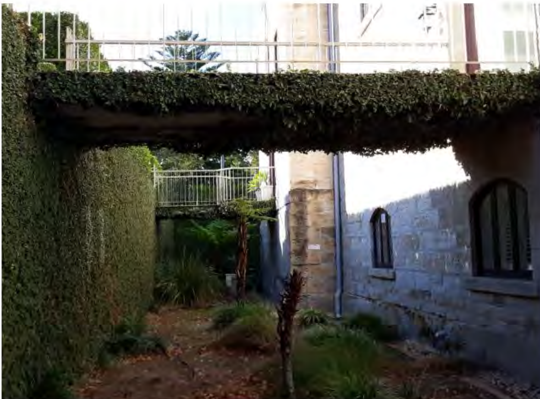
Image 2.8. Lower north façade showing sandstone cutting wall at left and bridges to entrances of the building. The bridge at the front gives access to 19 units in the main building while the bridge at the rear is used only by Unit 20, which occupies the entire three-storey eastern wing. (Source: BHHH, 2018)
